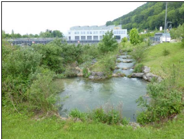
Ruppoldingen power plant (Switzerland), showing measures for fish passage and habitats: photo courtesy of Jukka Jormola, SYKE
