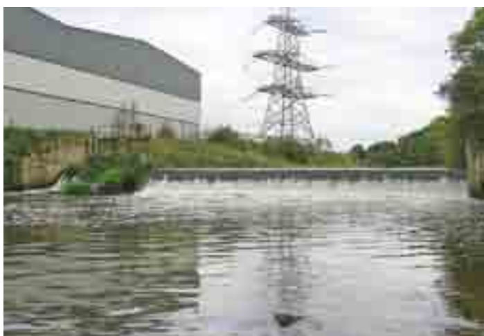
© Environment Agency Padiham Weir prior to works creating a total barrier to upstream fish migration – October 2005
