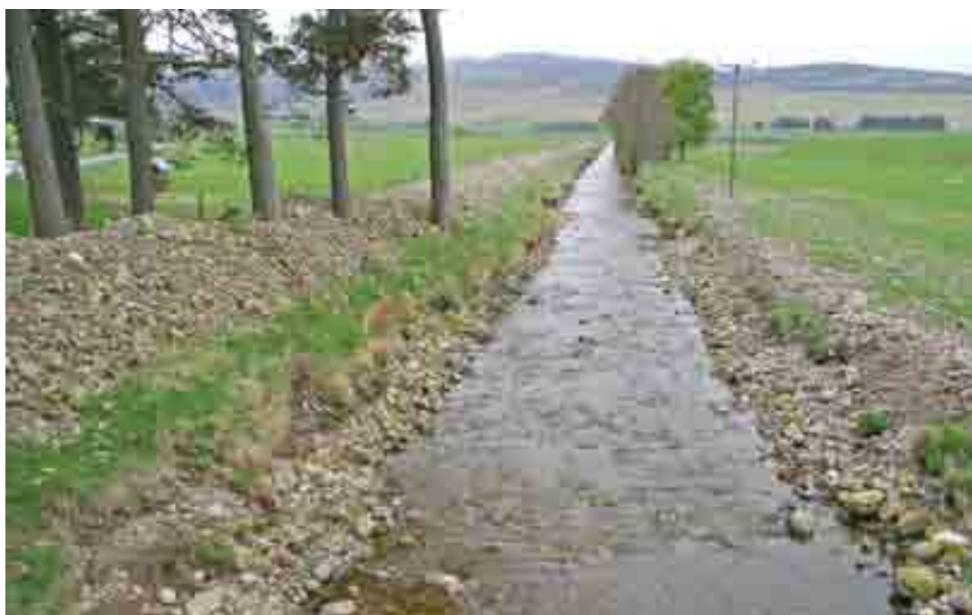
Dredged gravel forms an embankment on both banks. The channel runs in a straight line to the confluence with the River South Esk – May 2006
