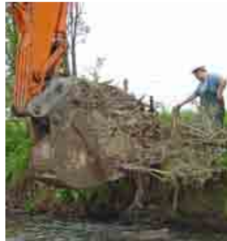
Installing root wad in bank– 2004
