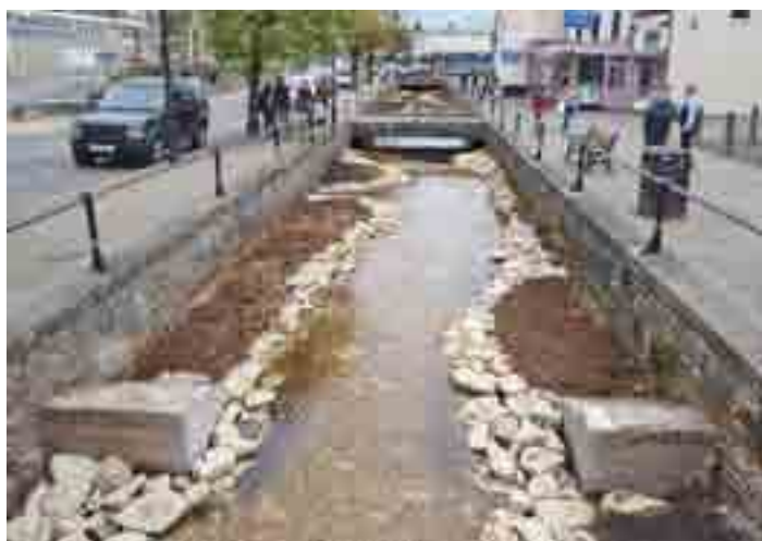
Two sides of the weir have been retained and incorporated into the berms – 2011
