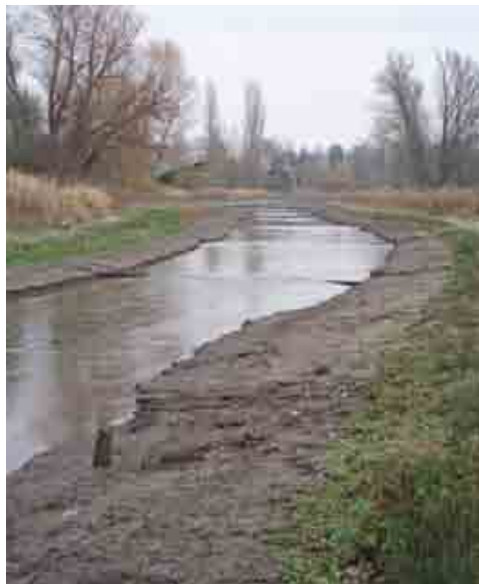
© Environment Agency The newly installed deflectors face upstream and concentrate flow. The old silt bed has formed new banks and has since been colonised by vegetation – February 2007
