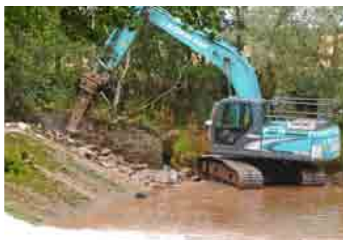
Initial breakout of the weir on the left bank – 2011
