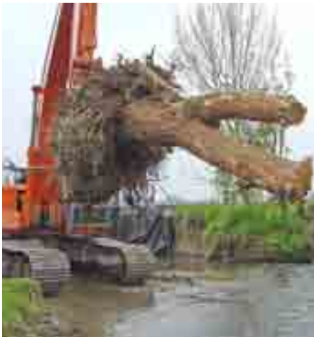
Excavator moving root wad into position– 2004
