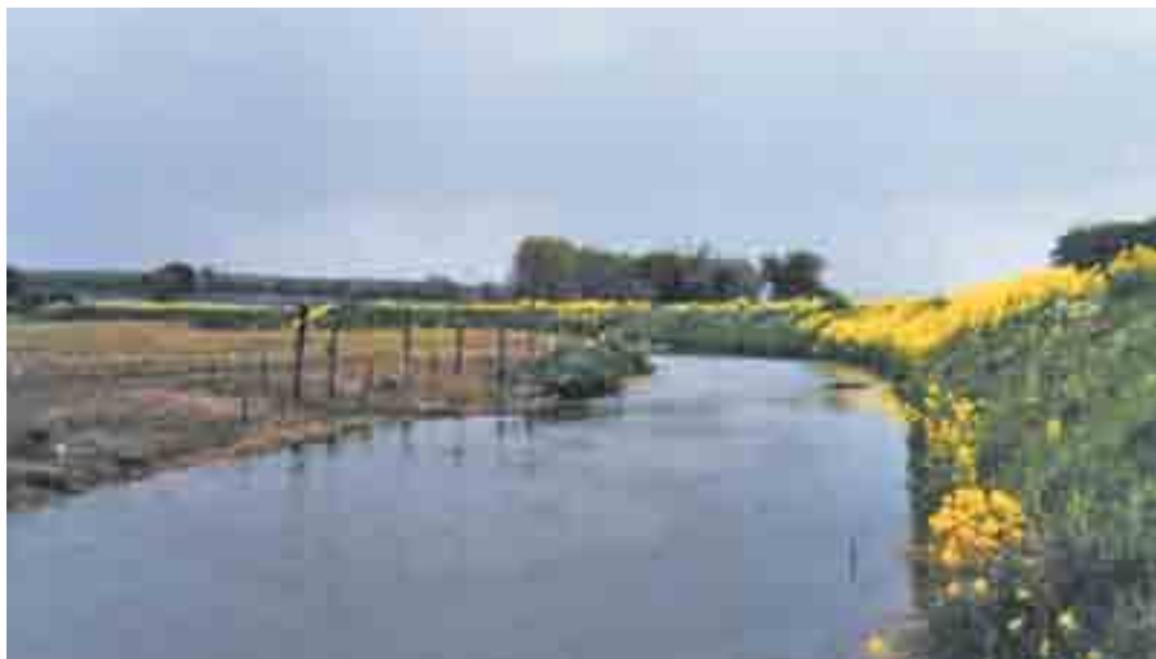
Removal of the left floodbank and marginal berm creation on the Great Eau at Withern
