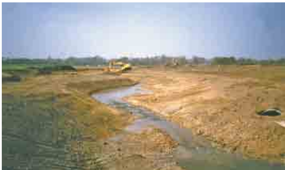
Looking downstream at the shallow bank slopes. The severed culvert still visible
