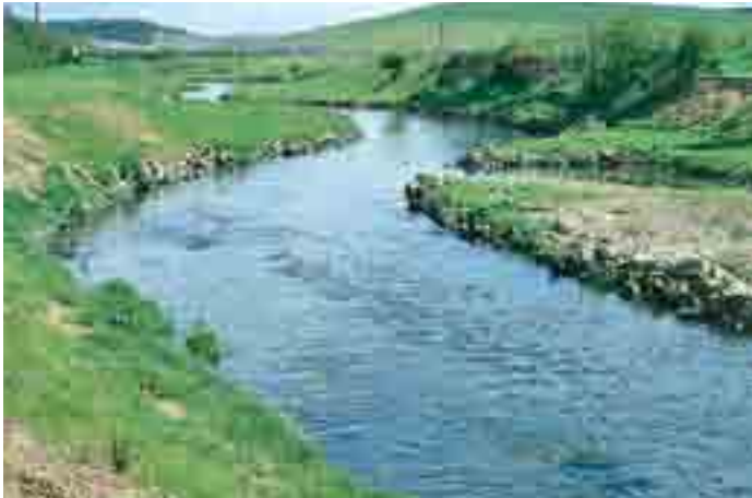
Narrowing increased velocities and created riffles used for fish spawning
