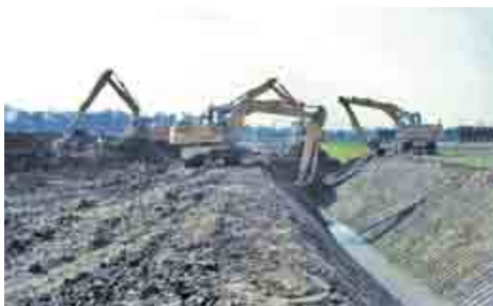
Relocating the IDB drain and set-back floodbank
