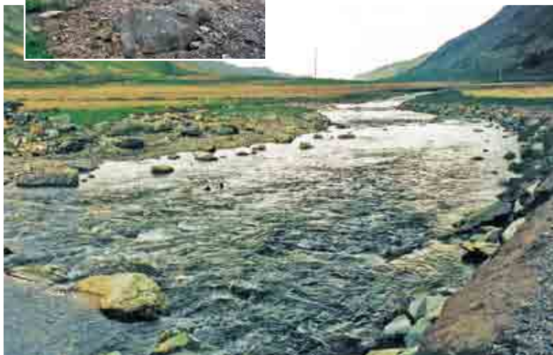
Restoration of boulder cascade, stepping stones and braided channel
