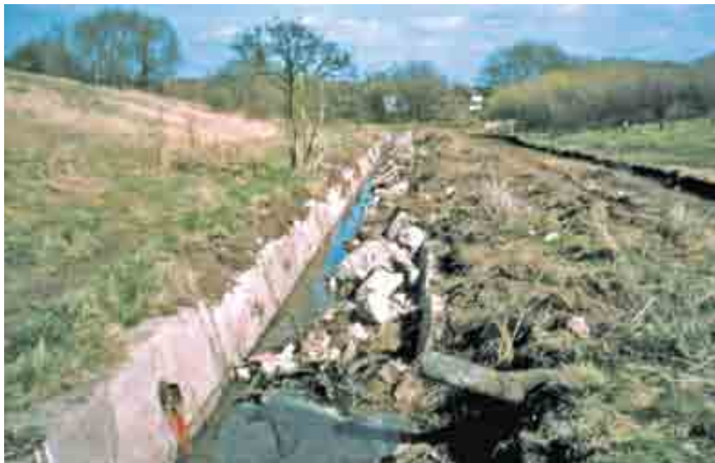
Concrete channel being broken up
