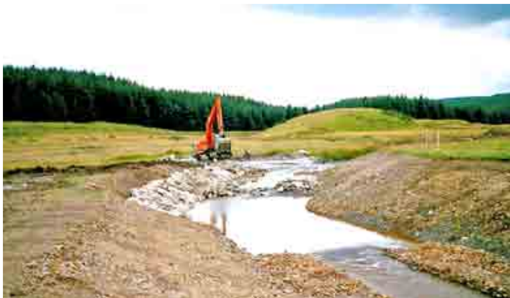
• a 1-2m wide depression was formed to create the low-flow channel, centrally on straight sections and towards the outside on bends ( Figures 11.2.2 and 11.2.3 ); • precautionary stone rip-rap was placed on meander bends to maintain the designed planform; • The bare banks were immediately hydroseeded with a grass mix to reflect the grassy moorland surroundings to maximise vegetation cover before the onset of winter.
