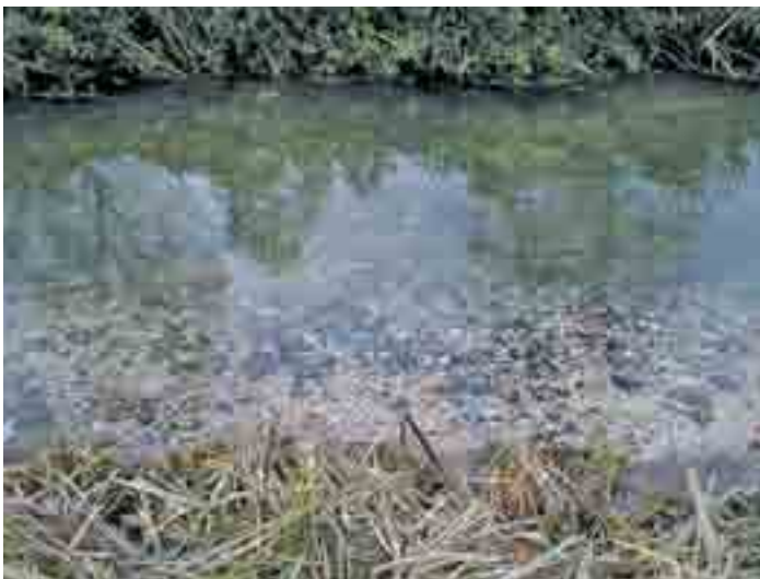
Flinty gravel used to narrow and raise the river bed
