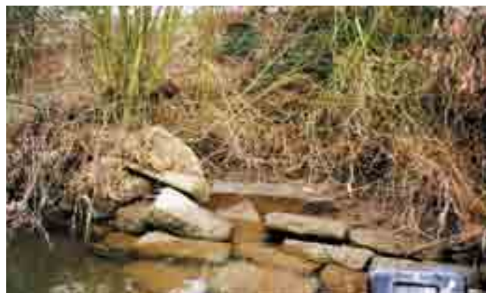
Failed section of bagwork at Clifton Lock Cut
