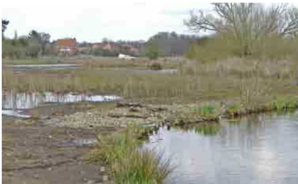
Erosion of the coir matting – April 2008
