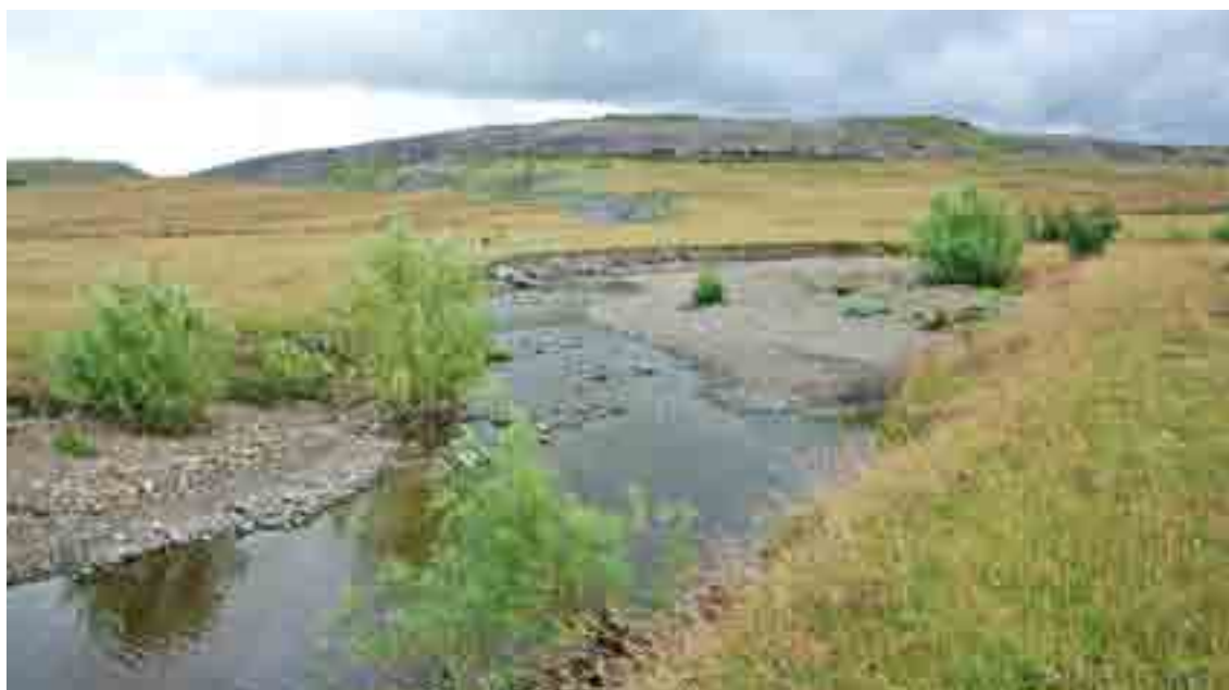
The channel realigned in 2004 after 7 years. Marginal vegetation has established and natural morphological processes are taking place – August 2011
