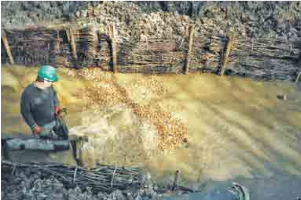
Gravel pumping in operation
