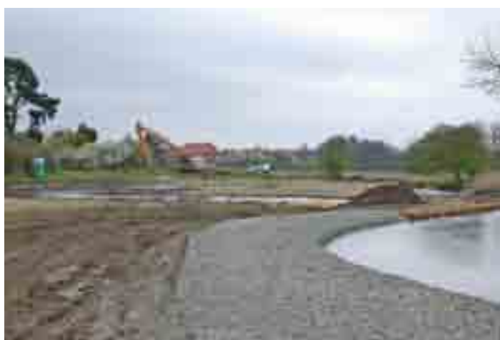
Same bank reinforced using blue clay – October 2003
