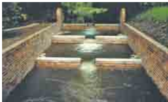
Mill weir and replacement fish-pass
