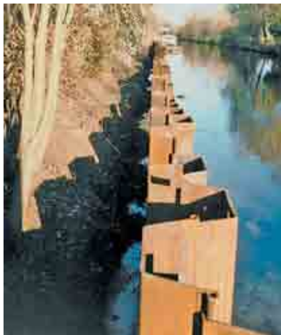
Initial sheet piling after bagwork removal, over existing trees
