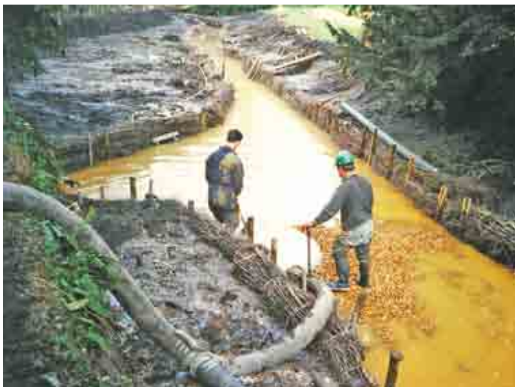
View of the wide dredged section, gravel being placed within the low-flow channel
