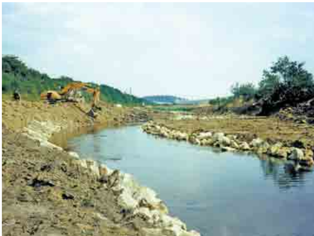
Placement of limestone boulders and berm back-filling
