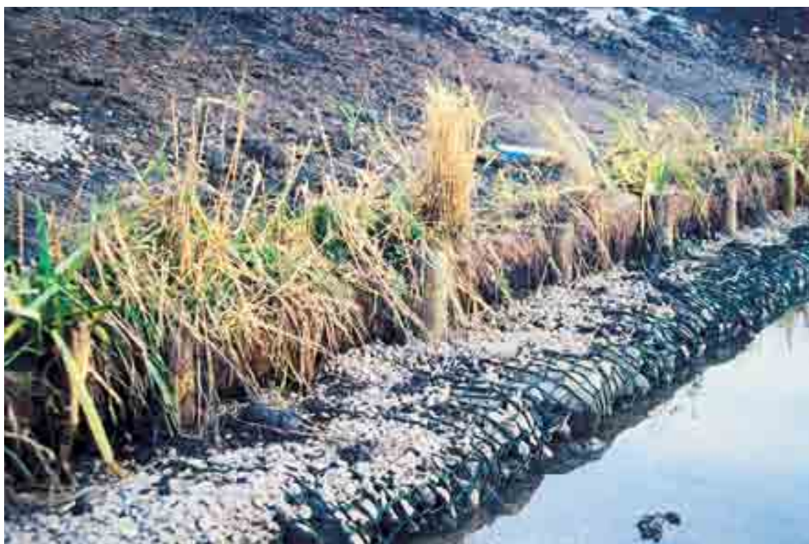
Transitional revetment at installation (water level artificially low in photo)
