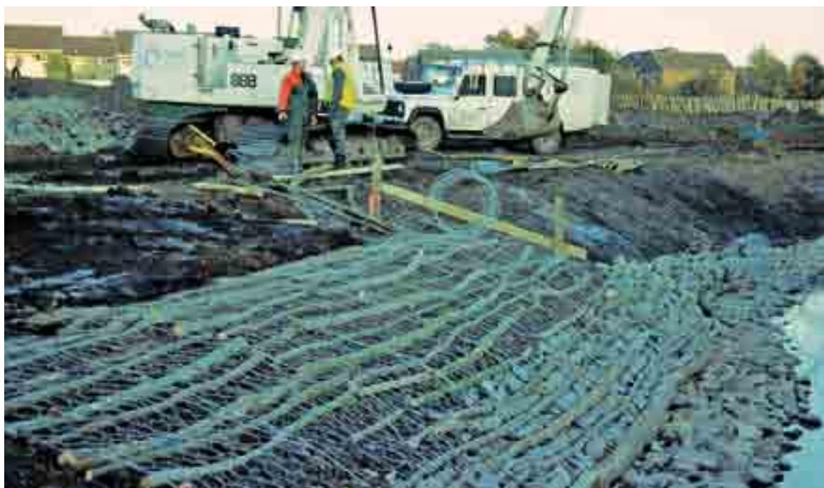
Mattress revetment under construction – October 1995
