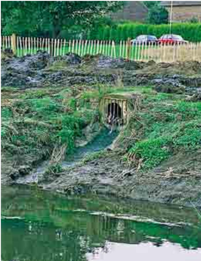
Typical outfall before replacement
