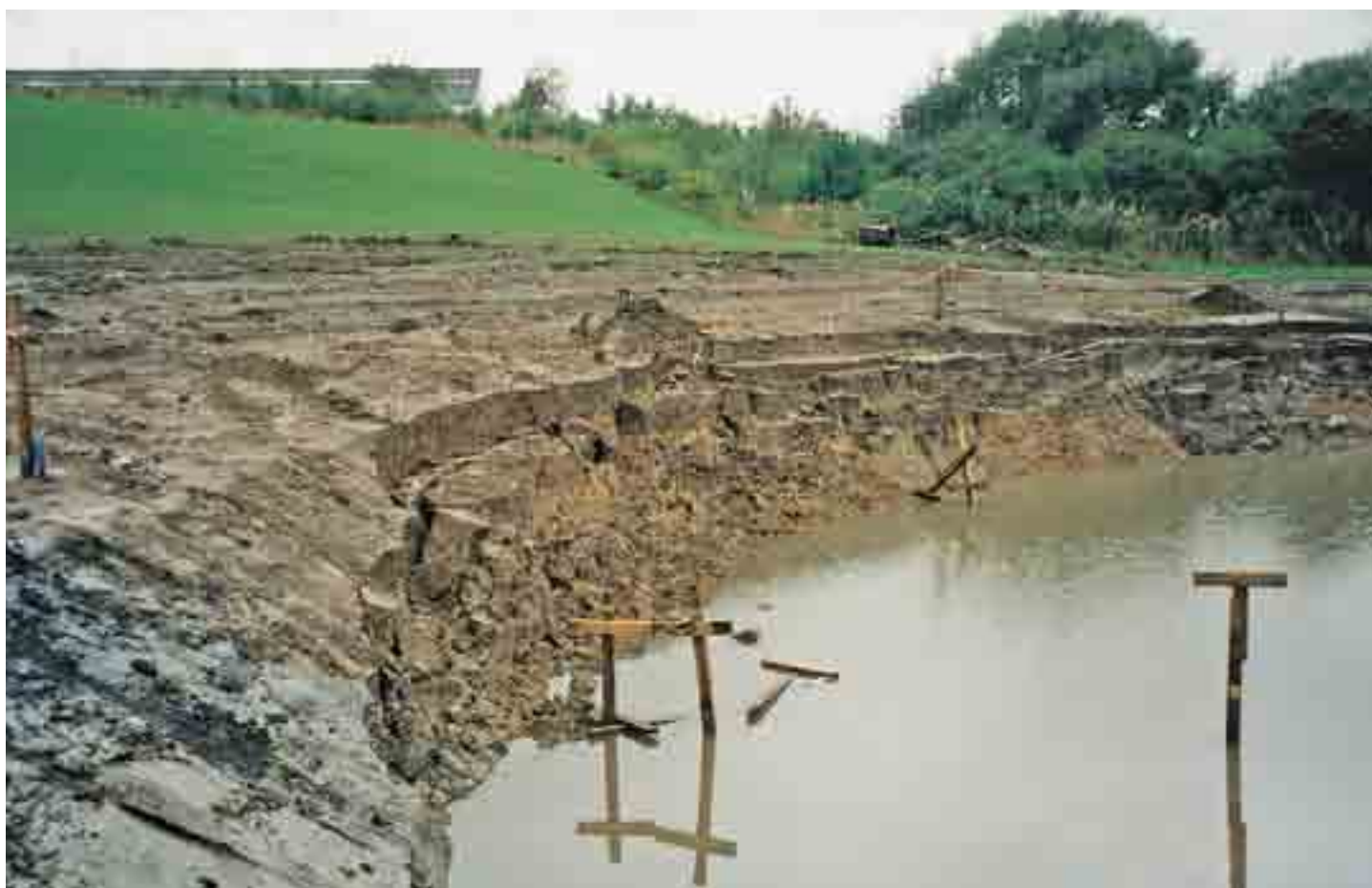
Slipped slope during work - September 1995
