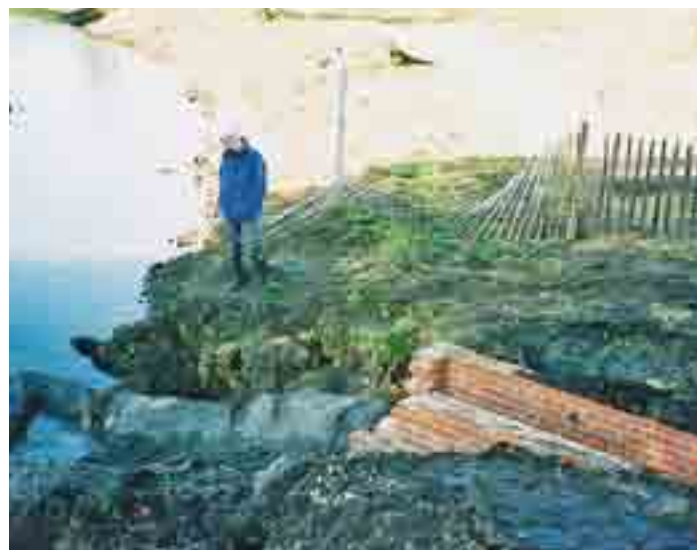
New outfall chamber under construction
