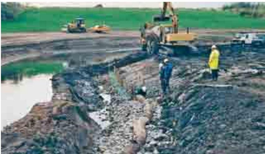
Log toe revetment during construction
