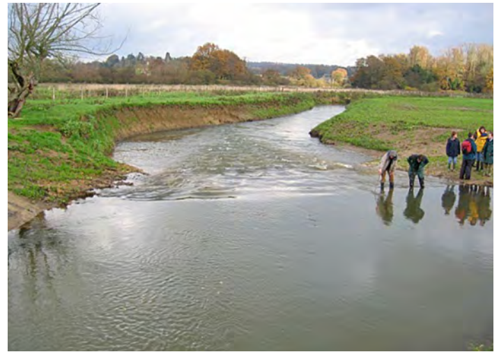
Bed check riffle and ford at entrance to the loop post-construction – 2004
