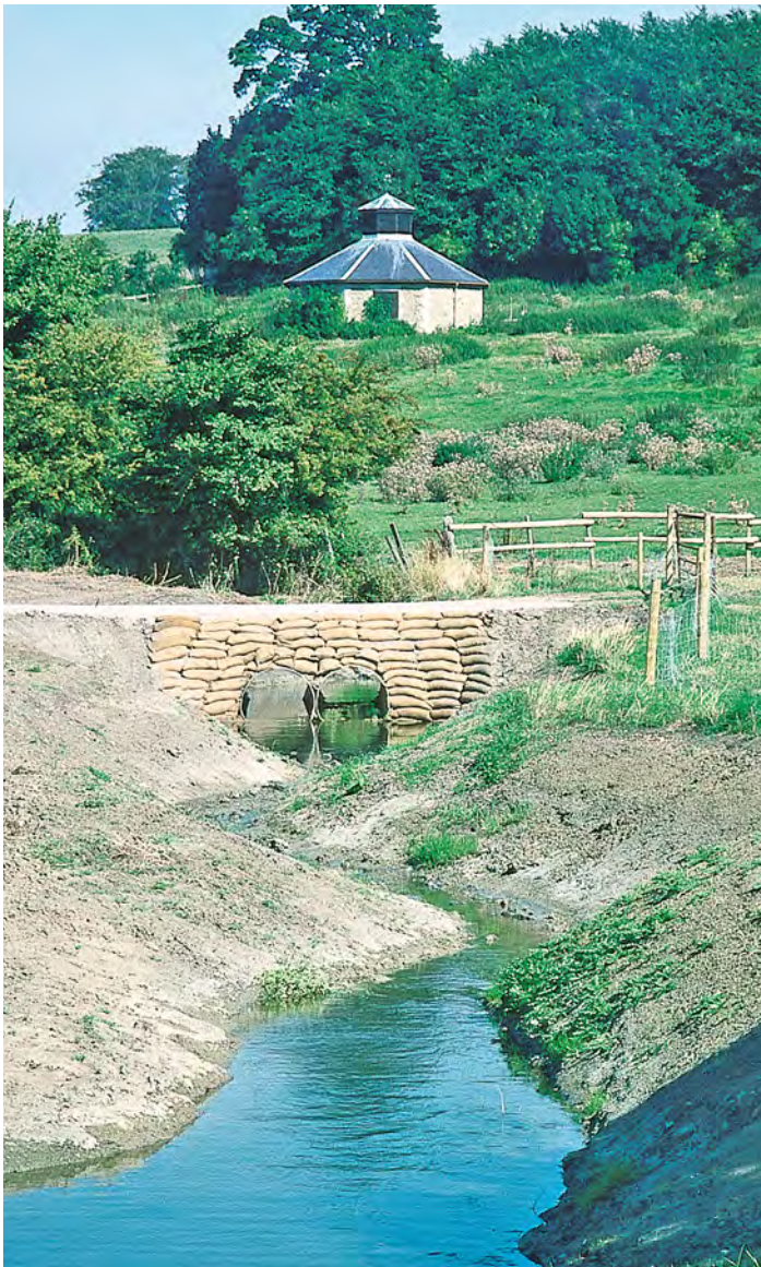
Flood drain crossing seen from bank of R. Cole. (bagwork wing walls incomplete)
