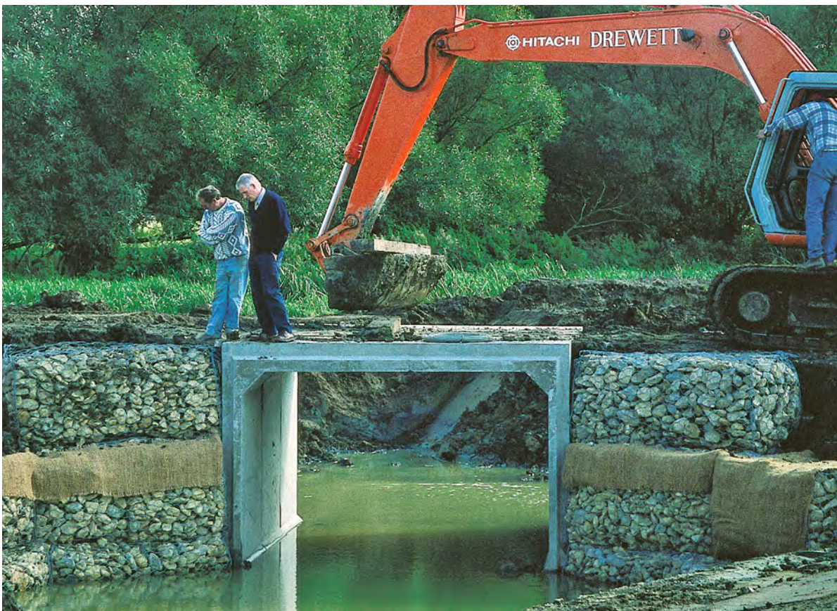
New concrete culvert crossing under construction
