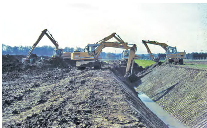
Relocating the IDB drain and set-back floodbank
