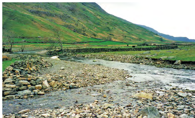
Restored bed levels and bank profile
