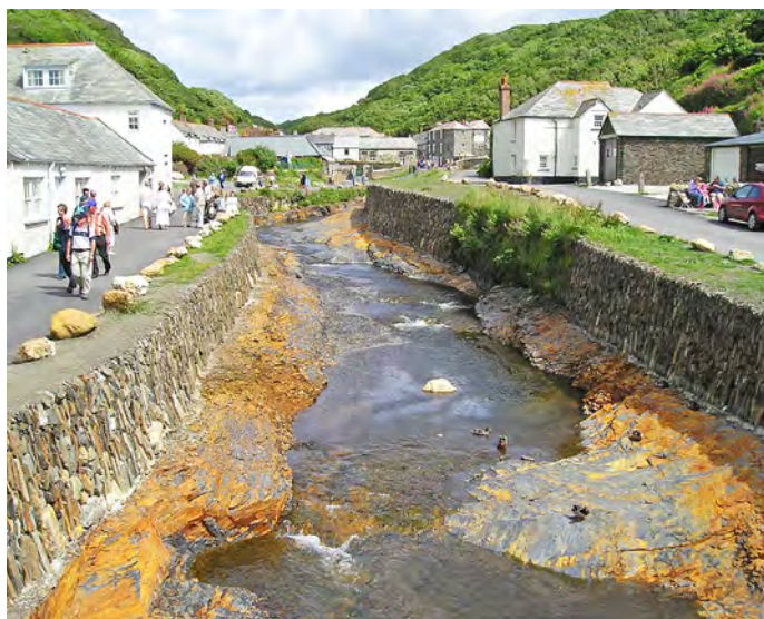
© Halcrow The low flow course had to be entirely excavated to best mimic millennia of erosion of a hard rock bed.
