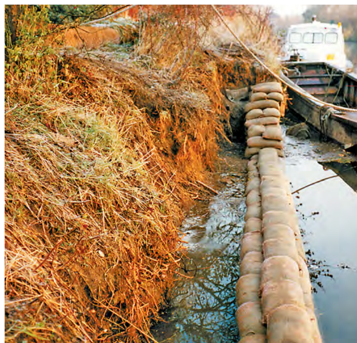
2 layer capping bagwork and tie-in to existing sheet piling
