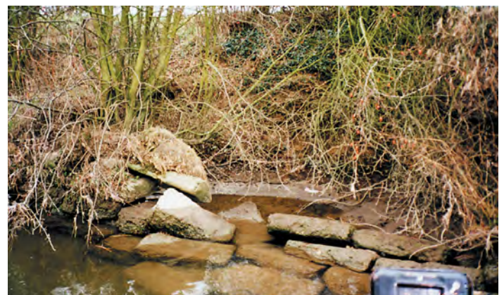
Failed section of bagwork at Clifton Lock Cut
