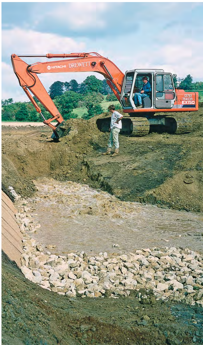
Construction of coir matting revetment – river being released
