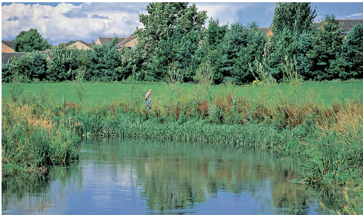
Log toe revetment three years after construction
