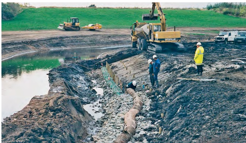
Log toe revetment during construction
