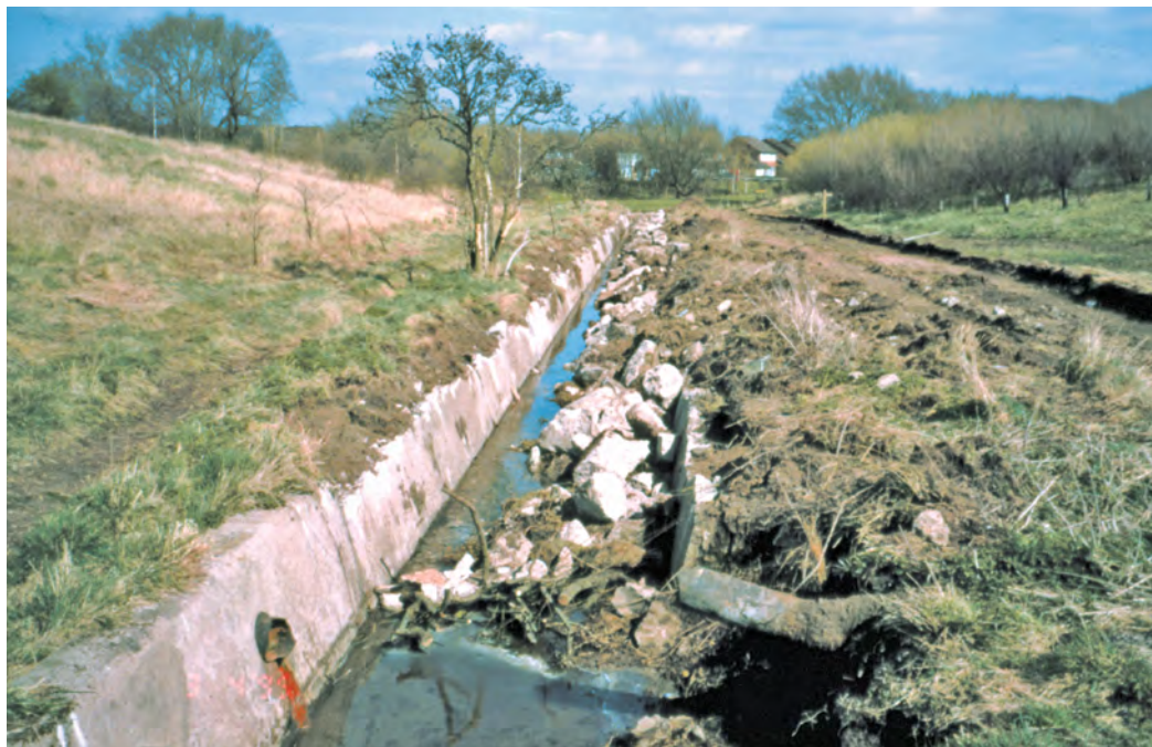
Concrete channel being broken up
