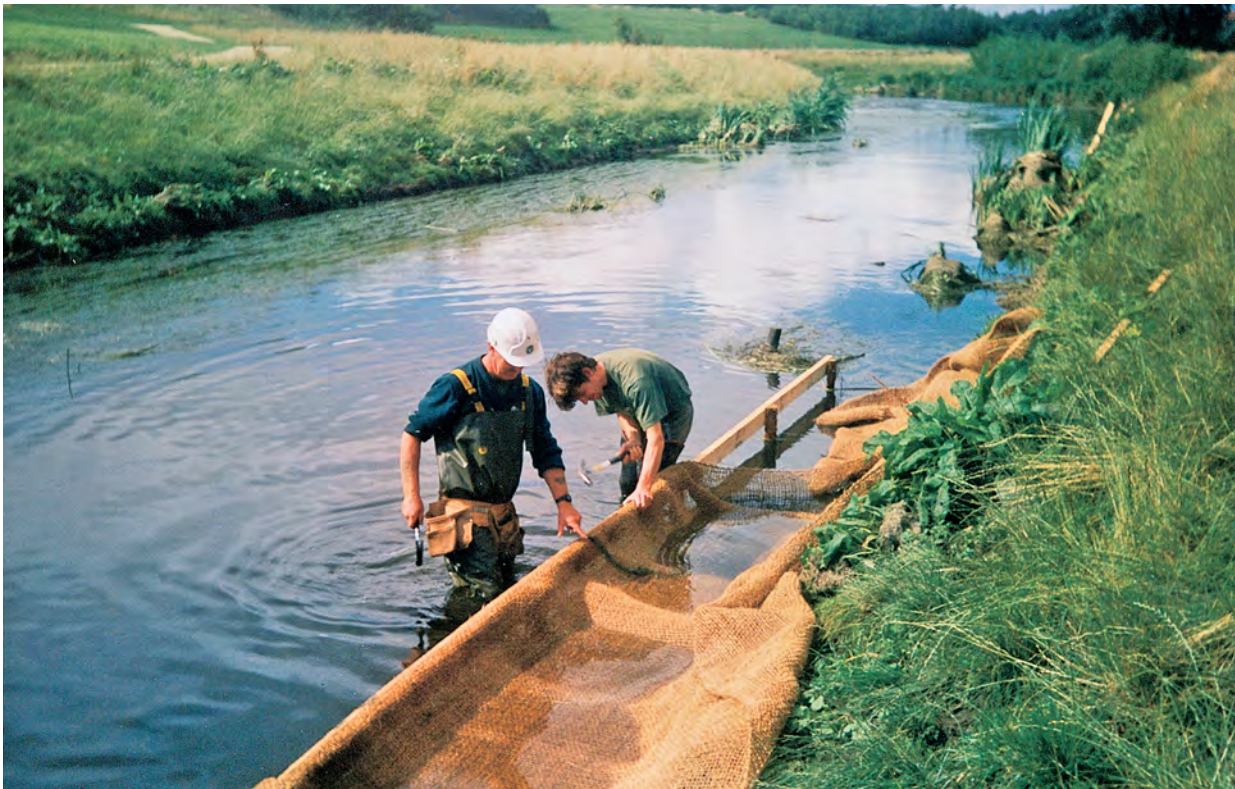
Attaching coir matting to create Type A ledges on River Skerne
