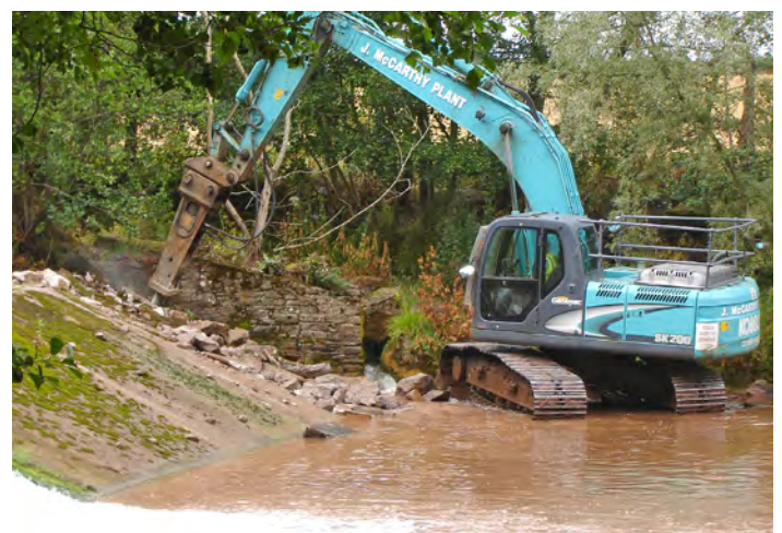
Initial breakout of the weir on the left bank – 2011
