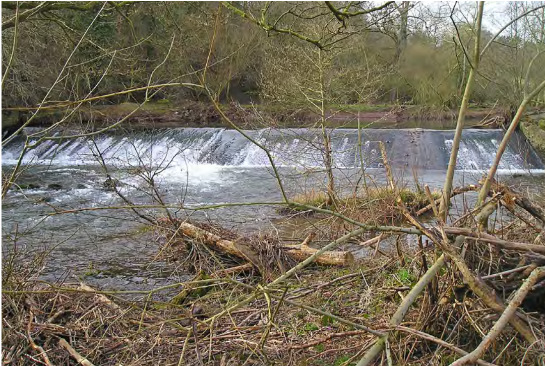
The 2.6m high Kentchurch Weir prior to removal – 2011
