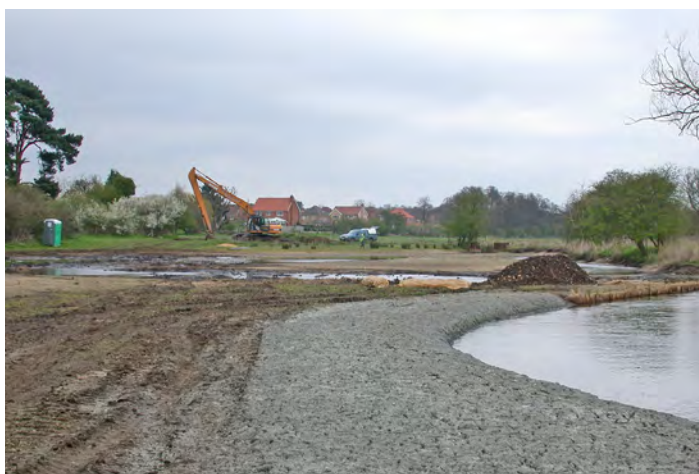
Same bank reinforced using blue clay – October 2003
