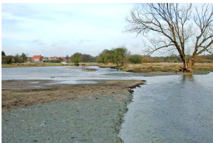
Breach of the reinforced clay bank – March 2004
