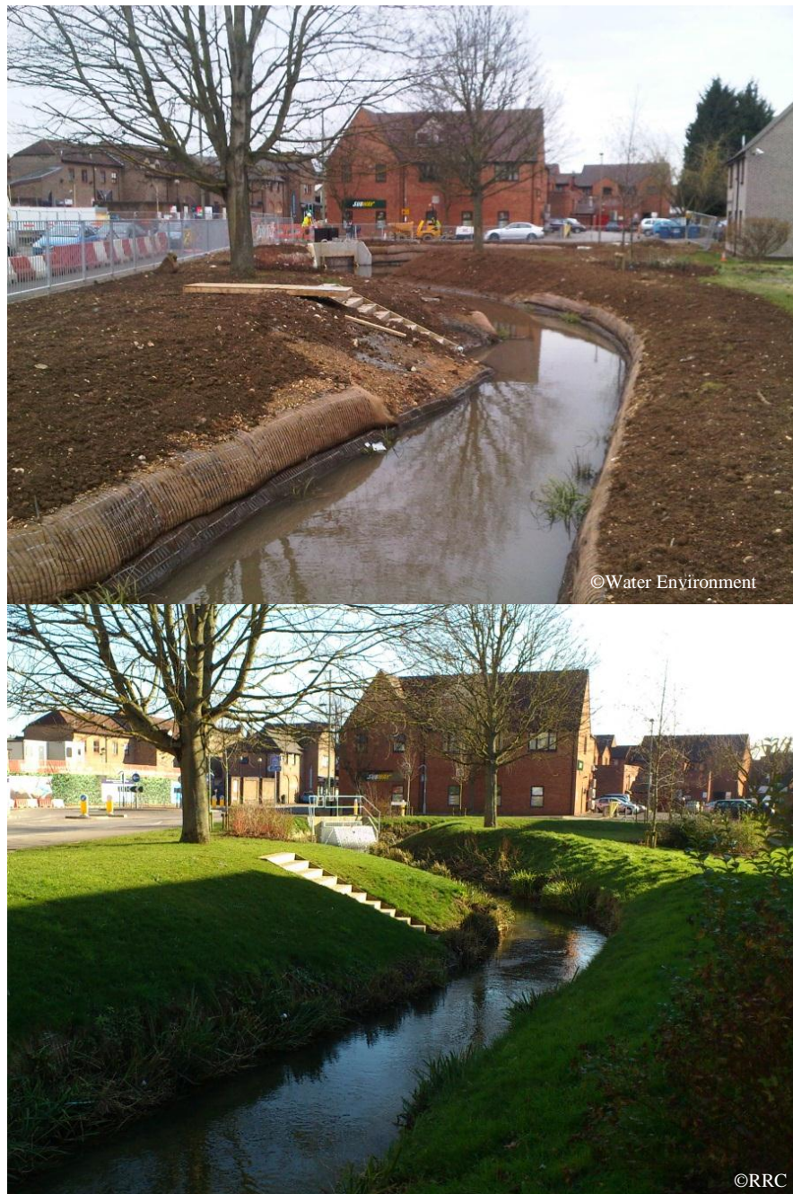
Figure 2: The channel diversion during construction (top) and 2 years on.
