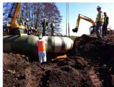
connecting the channels with siphon pipe
