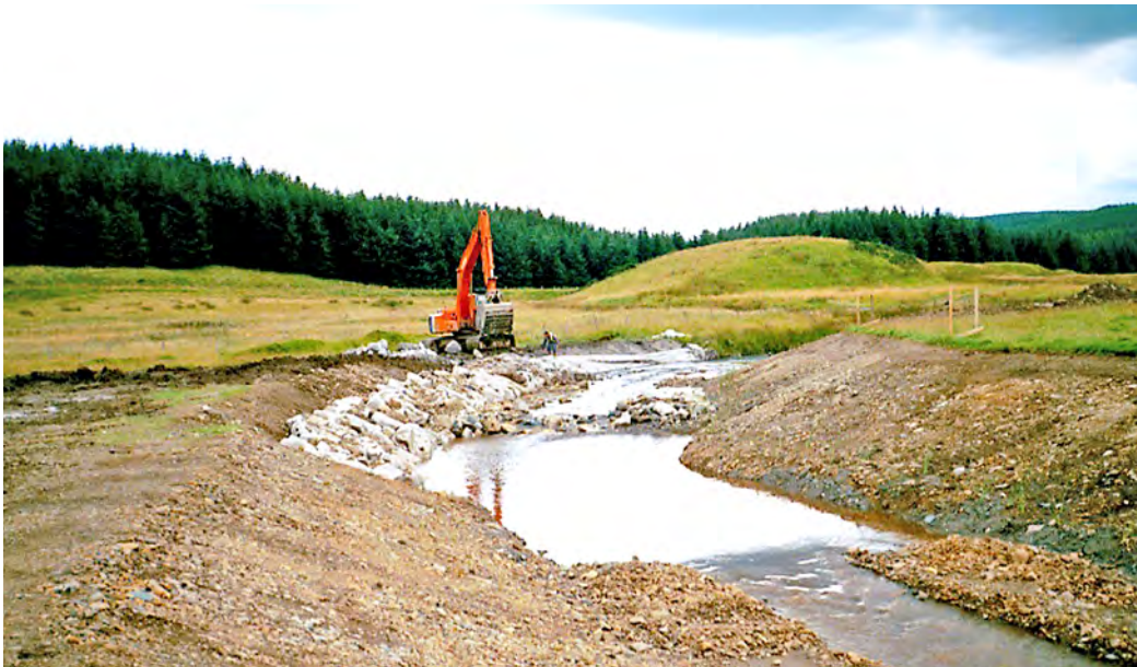
The 'constructed' run-pool-riffle sequence
