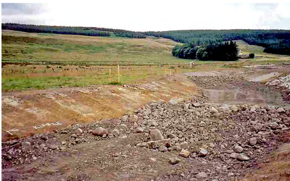
Shaping the new channel within the clay lining
