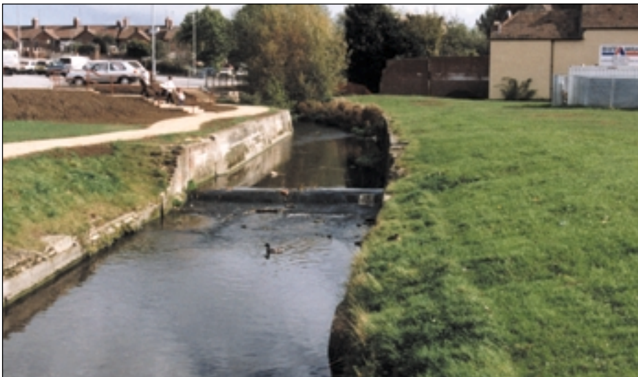
The river and weirs before construction
