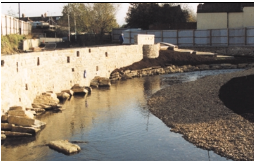
Gravel margins and seeded soil form the shallow banks opposite 'rocky' walls
