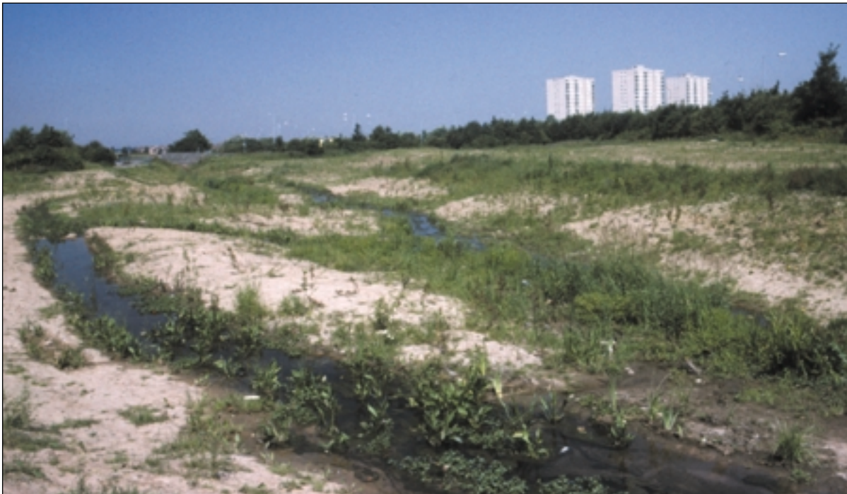
The excavated 'floodplain' area
