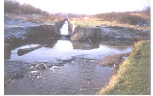
Yardley Brook prior to restoration works
