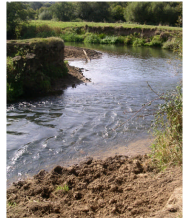
Stone riffle downstream of the loop to prevent acute gravel scour.
