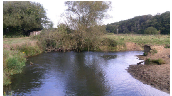
Downstream end of Shopham Loop with the cut blocked.
