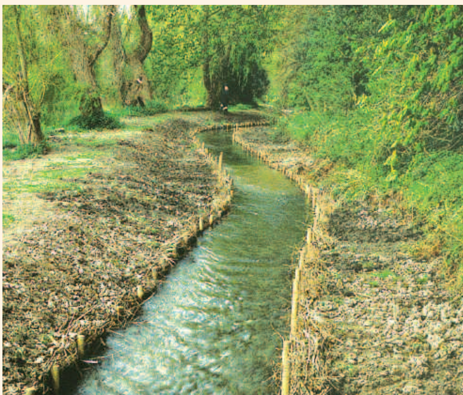
River channel narrowed using faggots (post-project, 1994)
