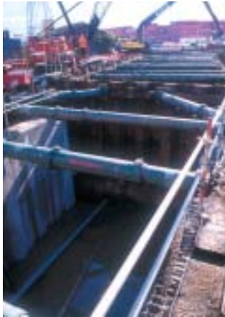
Culvert under construction
