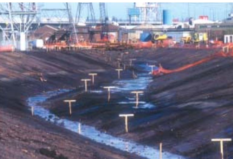
Dagenham Brook – construction of realigned channel
