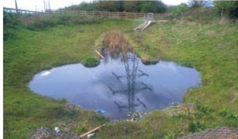
Retention pond – completed
