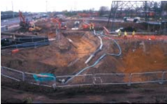
Retention pond – under construction
