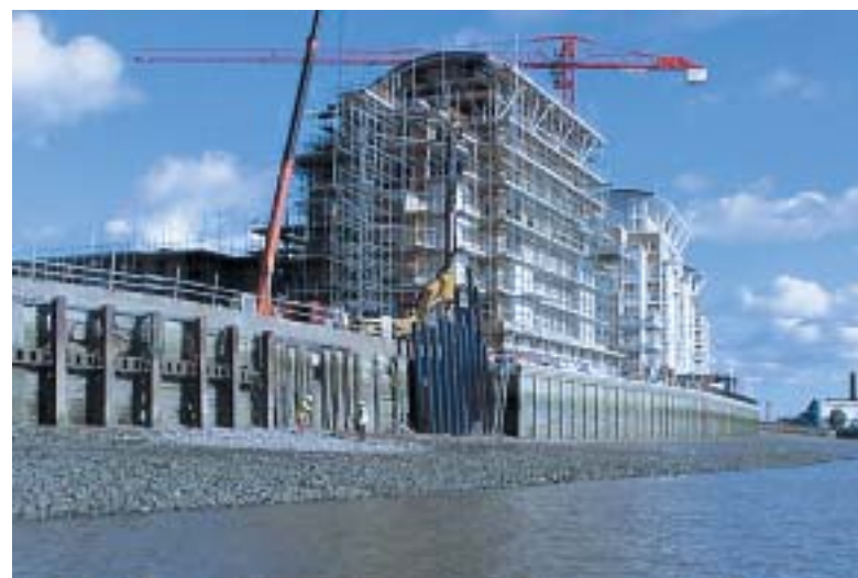
New flood defences under construction
