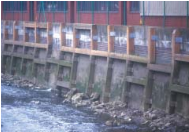
Mill Wharf – renewed flood defences
