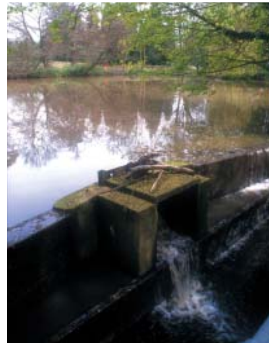
Temple Pond – overflow weir
