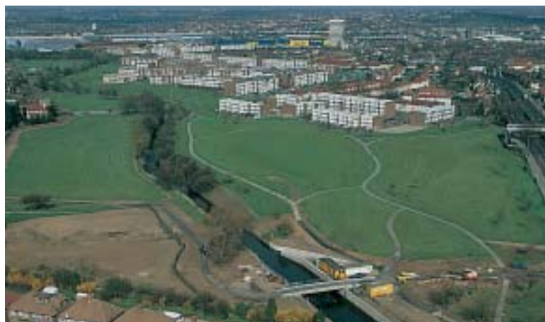
Tokyngton Park – aerial view
