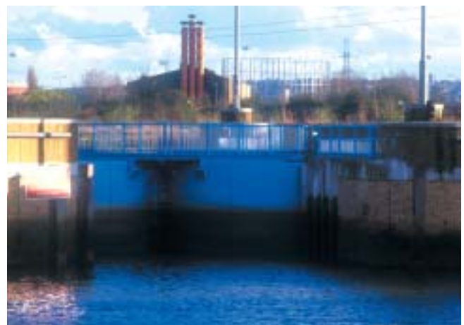
Barking Barrage – downstream of enhancement sites
