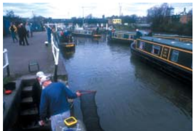
Brentford Lock – currently being redeveloped
