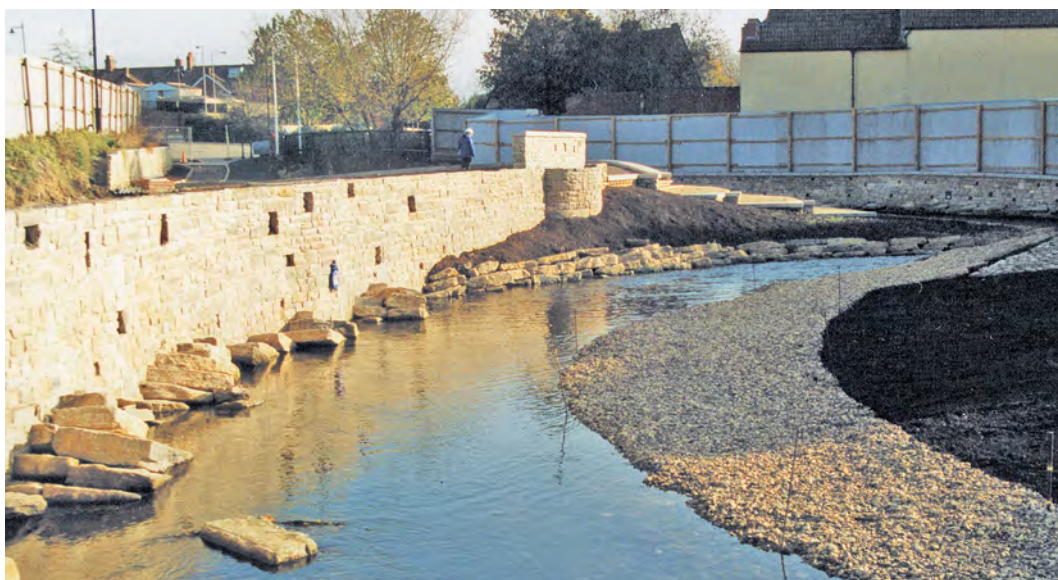
Gravel margins and seeded soil form the shallow banks opposite 'rocky' walls
