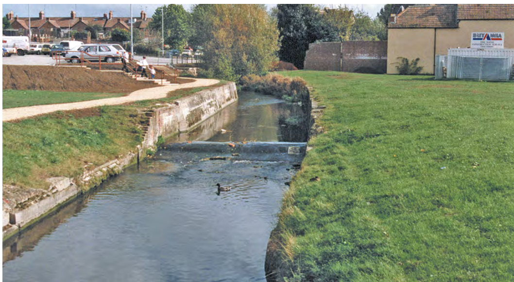
The river and weirs before reconstruction
