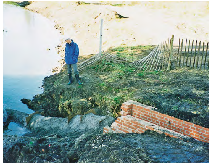
New outfall chamber under construction
