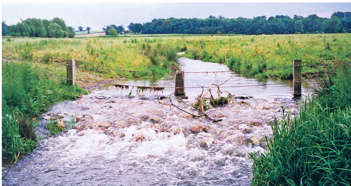
Weir and rock apron
