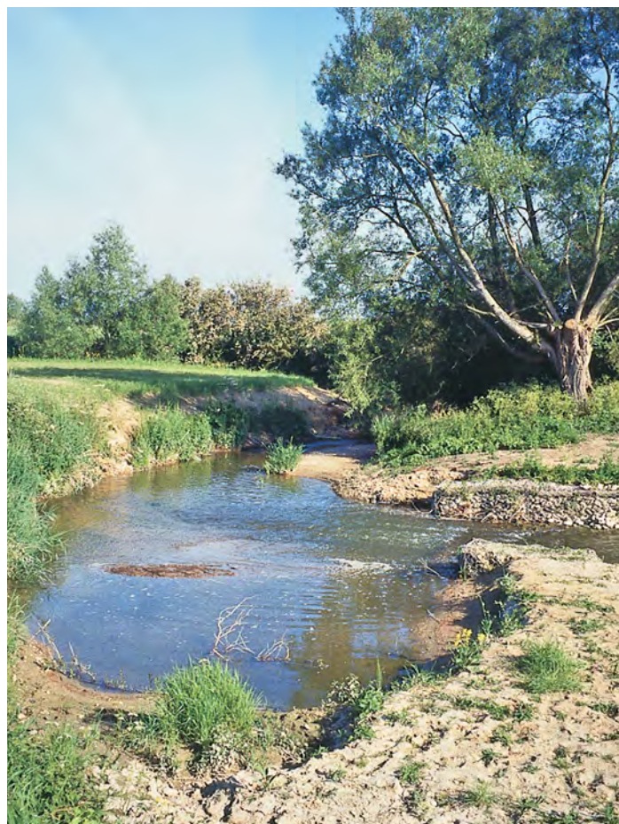
Gabion weir and pool
