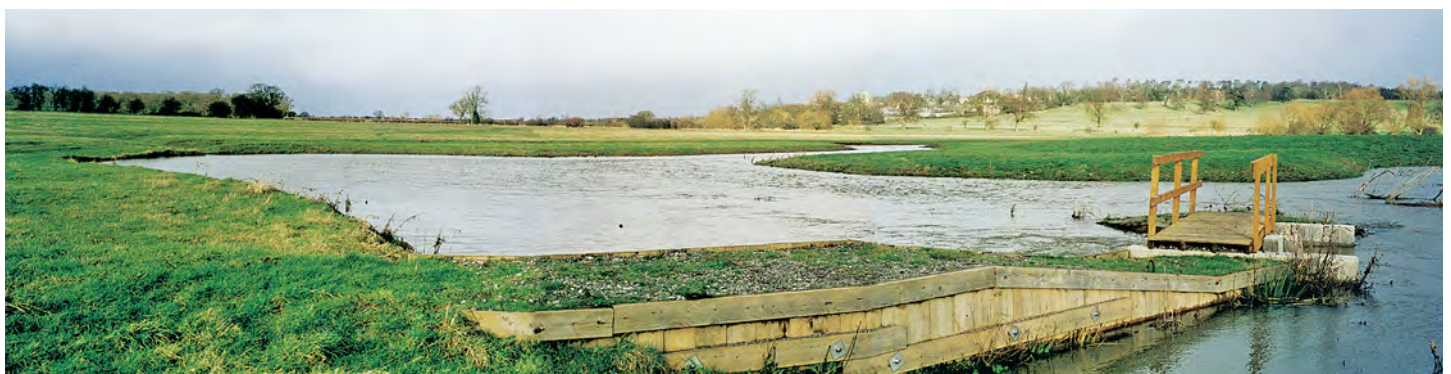
Flood filled channel downstream of bifurcation weir
