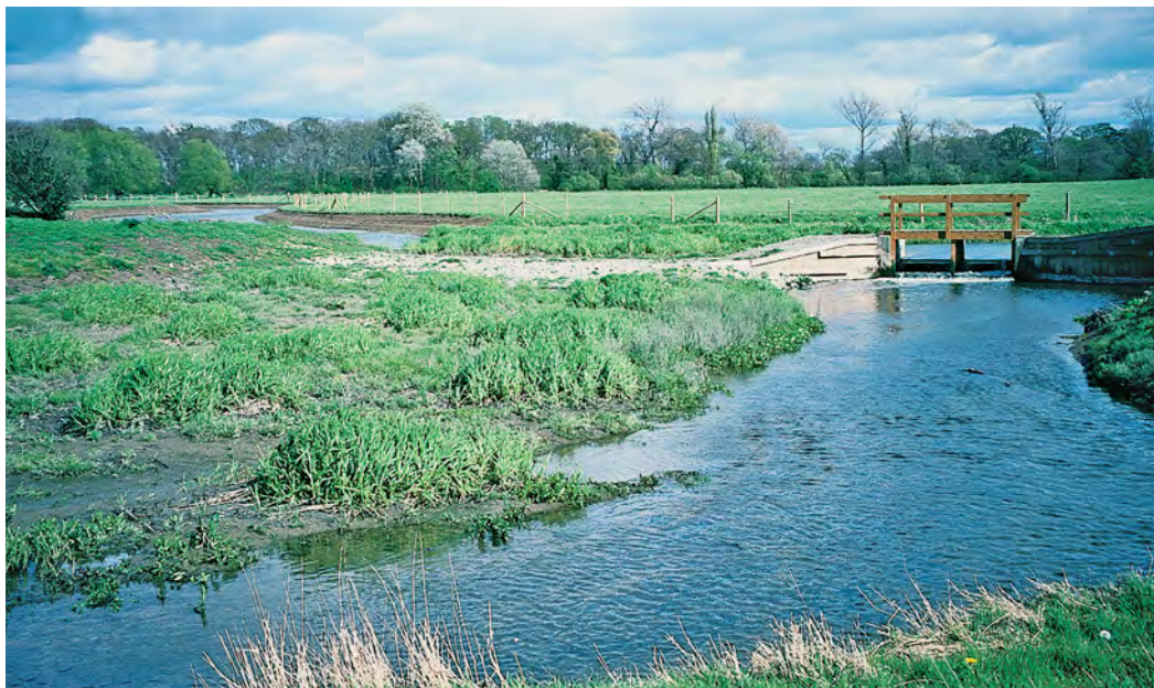
Spillway alongside bifurcation weir – April 1997
