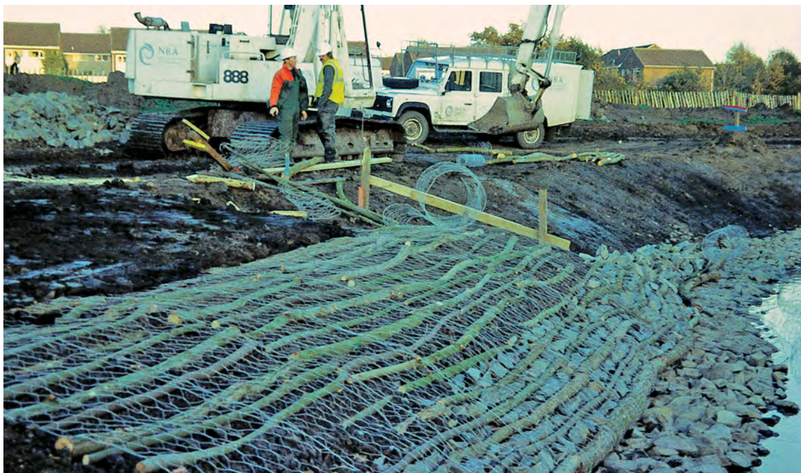
Mattress revetment under construction – October 1995
