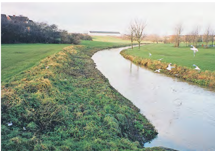
View downstream before deflectors constructed
