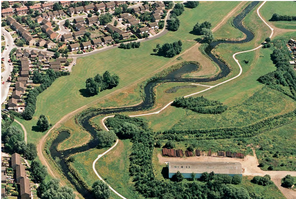
Completed meanders – Summer 1997
