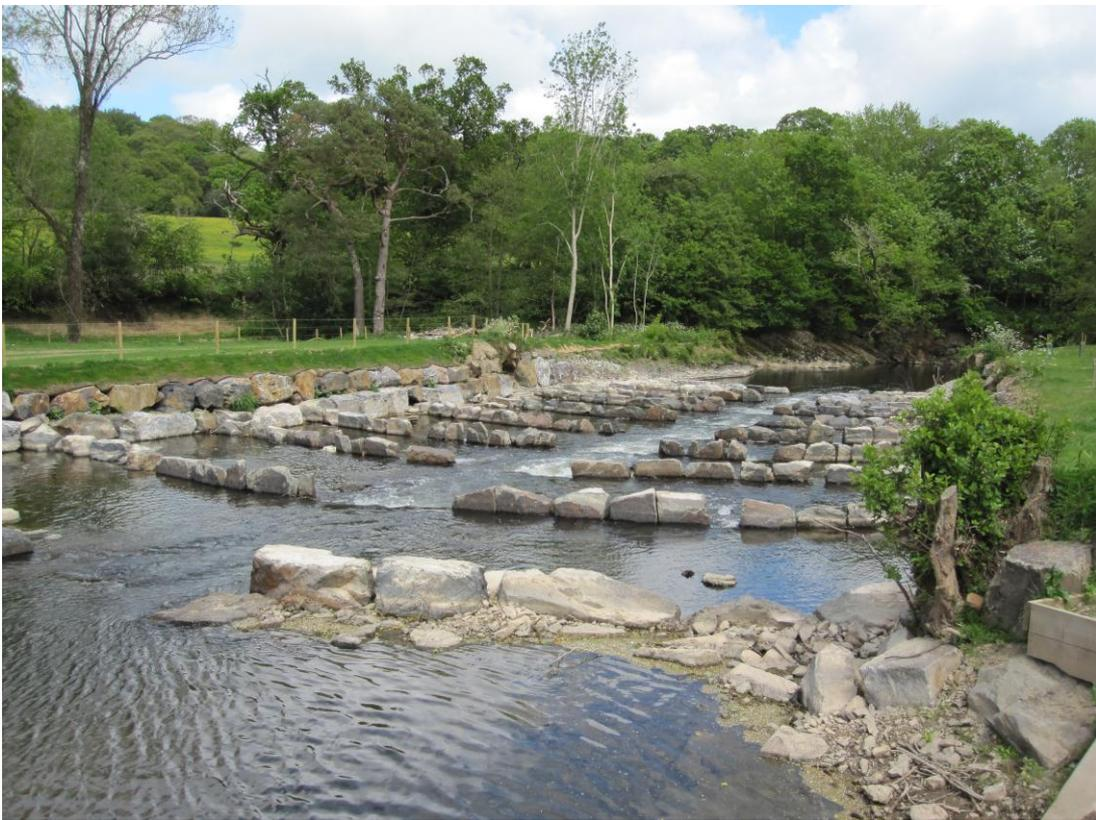
AFTER: The old weir was removed and replaced by a natural pool and riffle system, easily passable by fish.
