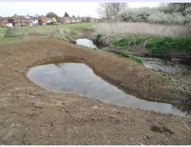
Graded backwater constructed to diversify river habitat. Graded to prevent fish being trapped at low water levels.
