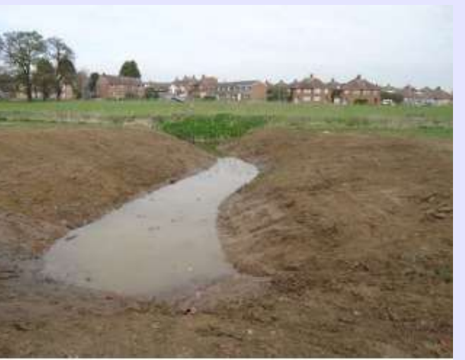
Further backwater constructed off main river channel
