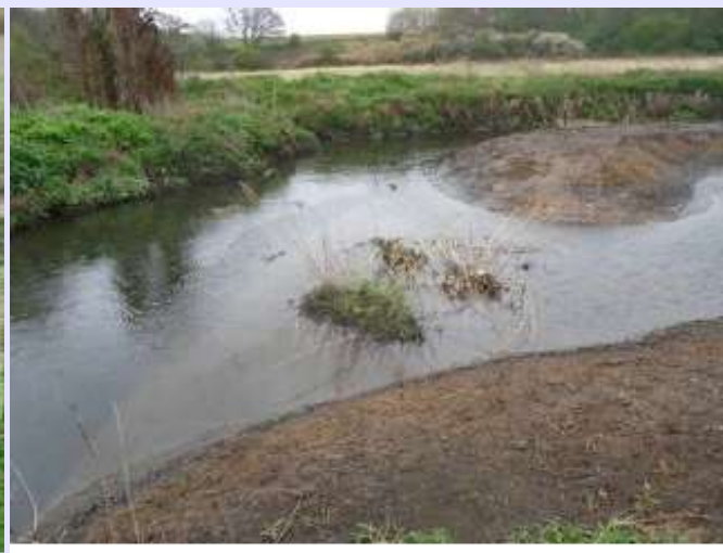
Island created by creating shallow shelf (depth of shelf just visible). Reeds placed back in channel to encourage growth
