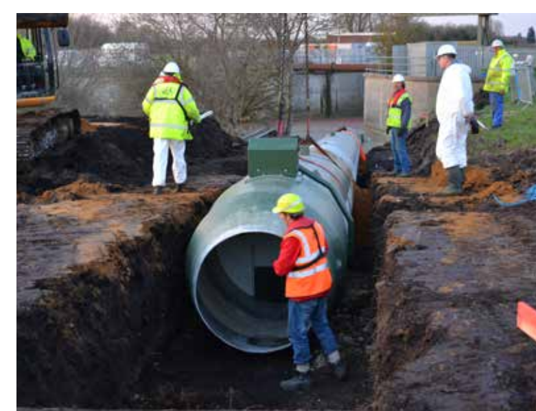
lowering siphon section into floodbank
