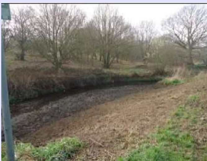
Lowered existing slumped bank material to summer water level
