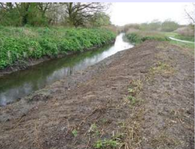
Berm created for flood protection to public footpath
