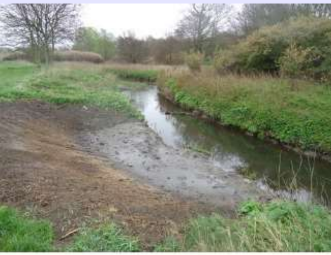
Shelf created to near summer water level increasing flood storage
