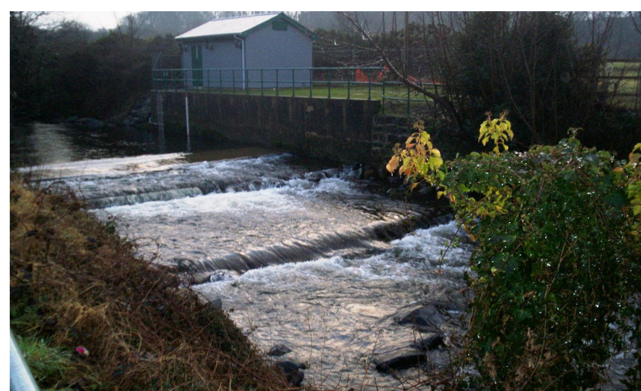
Rock ramp downstream of a gauging weir on Afon Gwyrfa.
