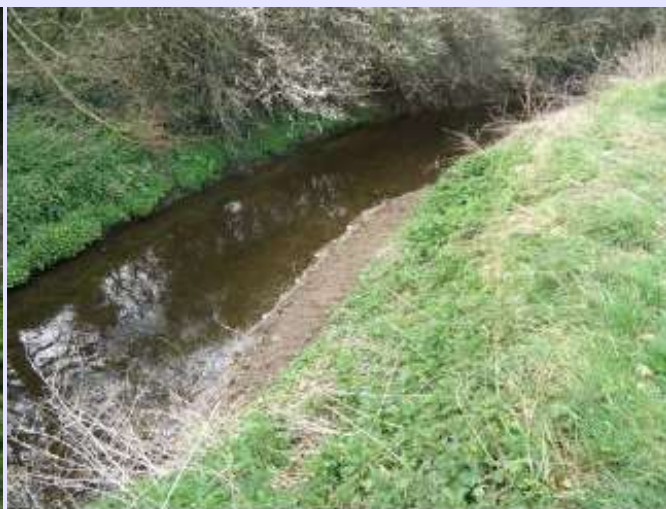
Berm created using faggots
