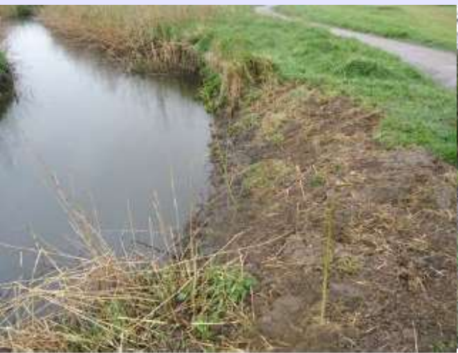
Soft engineering erosion control using wooden stakes
