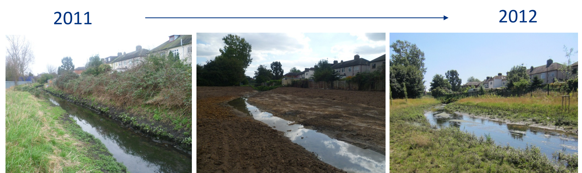
Transformation of the lower channel from an embanked straight channel to a meandering channel, reconnected with its floodplain (© LBBD/Nick Elbourne)
