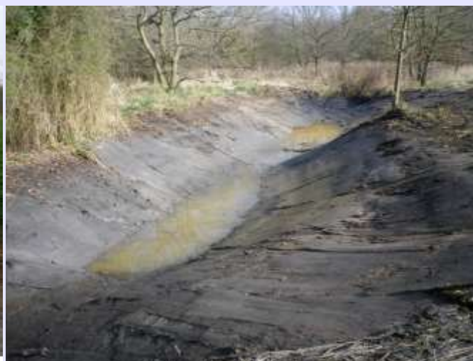
Construction of new attenuation pond
