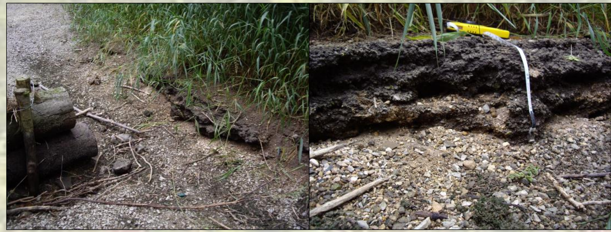
Figure 6 Two photos taken summer 2010 showing evidence of scouring either side of the fifth LWD structure in the reach.
