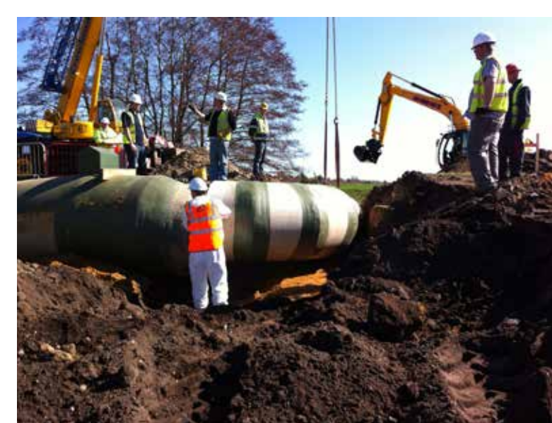
connecting the channels with siphon pipe
