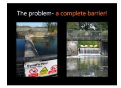
The Cam has been historically controlled at this location since the Domesday Survey with the current fixed crest weir and radial sluice gate constructed in 1949 to control discharge downstream and to retain upstream water levels for recreational and conservation.
