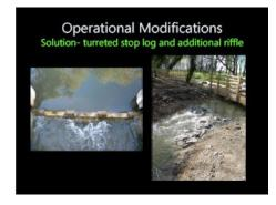
Solution- I cut three sections (450mm wide by 100mm deep) out of the retained stop log to try and resolve this. The head difference was reduced by c.100mm however the flow through the turreted log was still too high for Minnows to be able to negotiate the structure.
