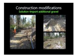
Solution-To form the channel to the dimensions as designed an additional mixed fill of claybound rejects, ranging from 20-100mm, and graded gravel 10-20mm was imported. This material was also used to infill areas which had become unstable during the removal of silts from the main channel. This provided the opportunity for shallow gravel margins alongside the main channel diversifying the habitat.
