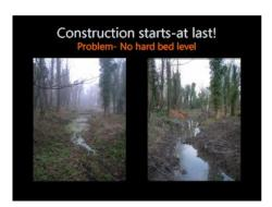
Problem- During excavation of the channel the hard bed level identified in the topographic survey was not found. This meant that the channel could not be formed as designed and that if constructed as is, the channel morphology and heterogeneity of flow characteristics would be lost the moment the pass became operational!
