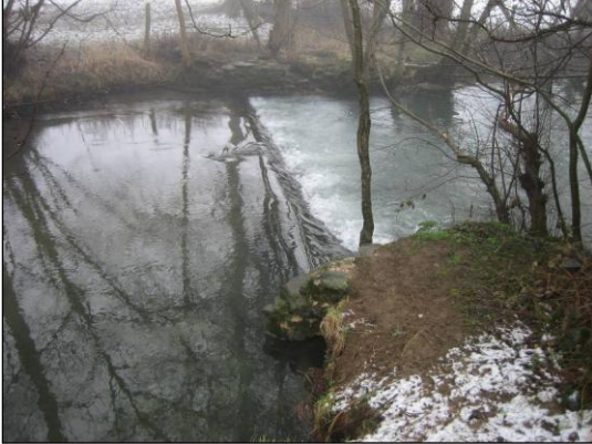
Figure 1 Example 1 - Unamed weir on the River Lugg, near to Prestigne (Powys) – Weir height approximately 0.5m, channel width at the weir 5m
