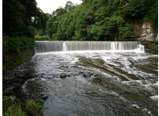
Figure 2 Example 2 - Peggies Mill weir on the Lower reaches of the River Almond (Cramond near Edinburgh) – Weir height 3.5m, channel width at the weir 30m
