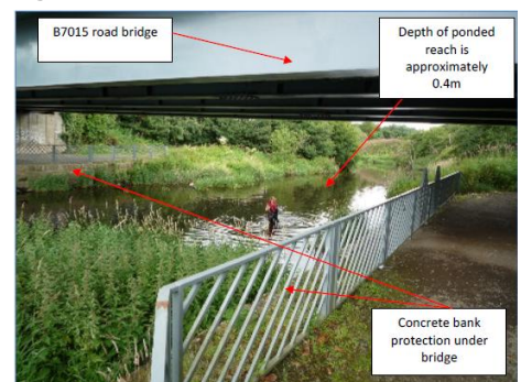
Figure 8 - B7015 road bridge 200m upstream from weir
