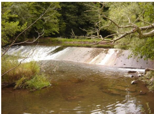
Figure 6 – Kentchurch Weir, River Monnow
